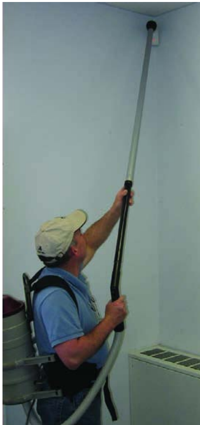
Use lightweight plastic extension handles when vacuuming walls
